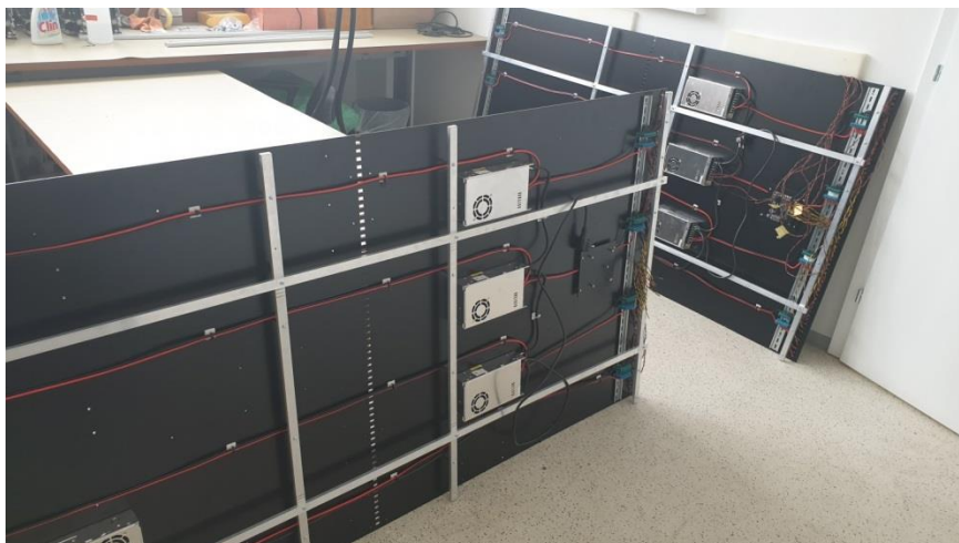
Figure 9. Segmented (Zig-Zag) Display Setup During the Build-Up
